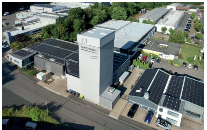
🌞 The company’s own solar power system is at the heart of Hartmann’s sustainable production strategy.
